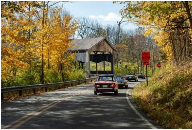
Heading south, we passed the Nixon Bridge, but did not cross it, hugging the west bank of the Little Miami instead...
