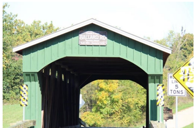
Ballard Road Bridge
